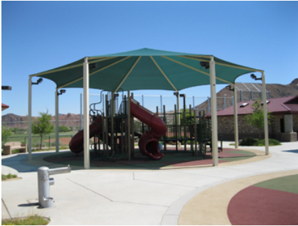
Tuscany Park, Henderson Nevada, Octagon Fabric Shade Structure. Courtesy USA Shade & Fabric Structures, Inc.
